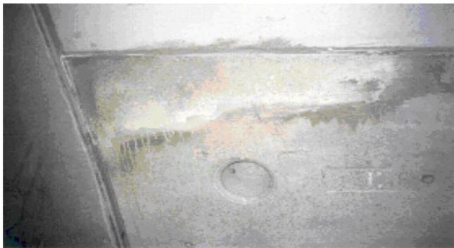
Figure 1. Repaired Concrete Tunnel Section
